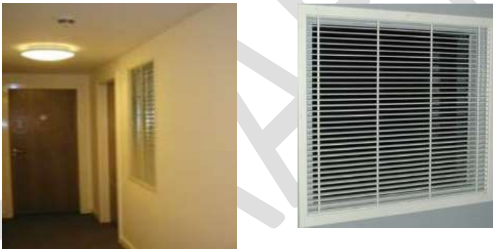
Figure 19 Corridor Automatic Ventilators to Smoke Shaft
