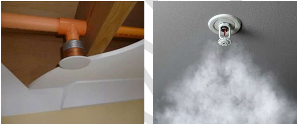
Figure 22 Concealed Sprinkler Head/ Sprinkler Head
