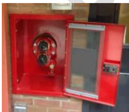
Figure 16(a) Inlet Breeching at exterior of building
