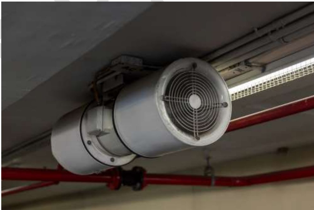
Figure 26 (a) Car Park impulse Ventilation System
