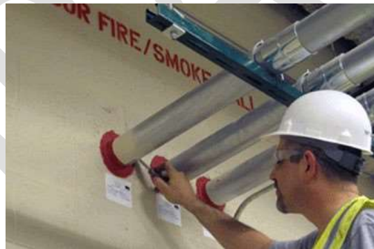
Figure 28 Fire Stopping of Pipe Penetration Wall
