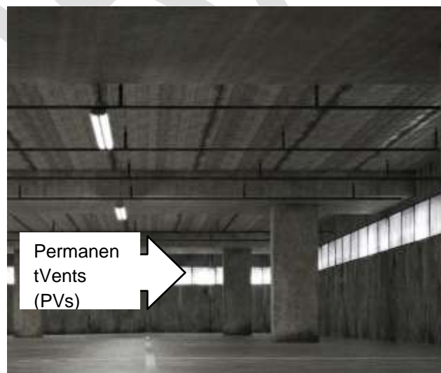
Figure 27 Car Park permanent ventilation openings to the external air
