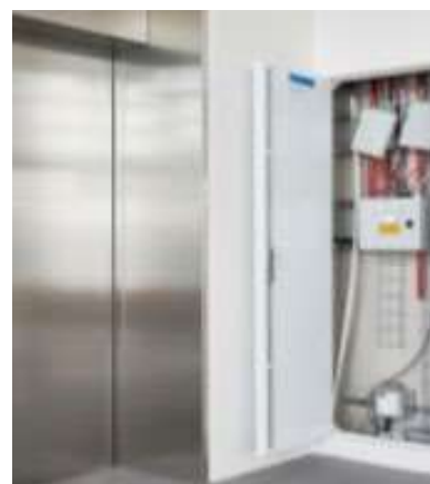
Figure 29 Service Risers in Common Areas
