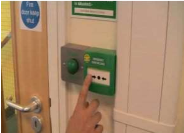
Figure 24 Egress Door with Door Release Device
