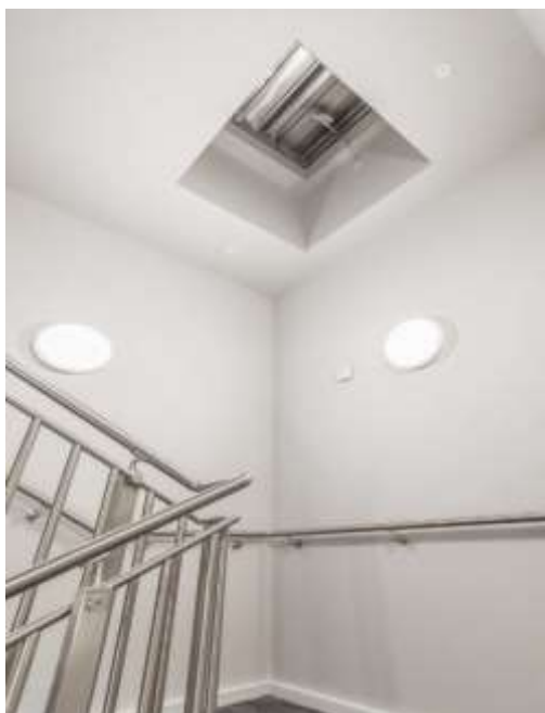
Figure 21 Roof mounted Automatic opening vent (AOV) and Controls
